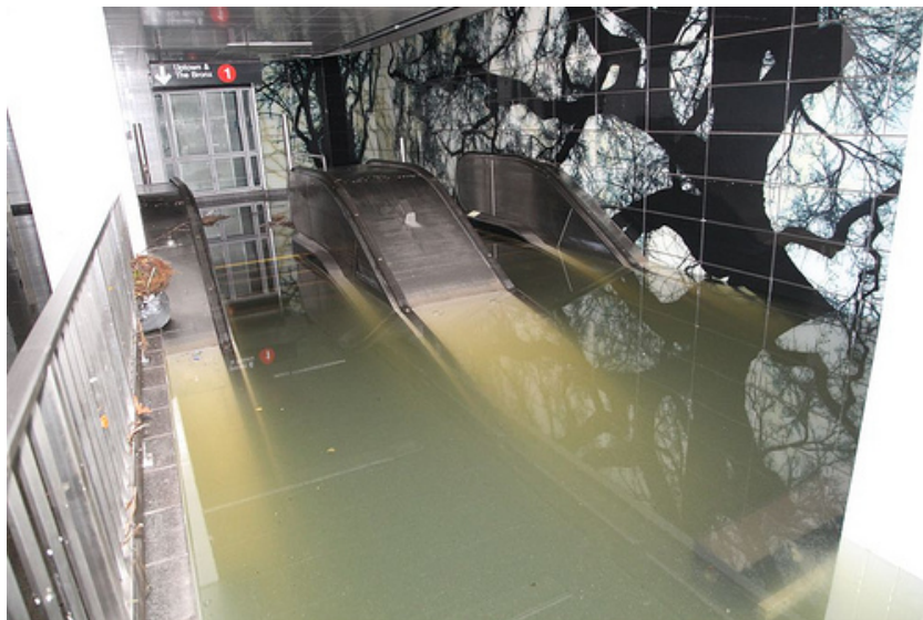
South Ferry subway station under water, the day after Hurricane Sandy (credit: MTAPhotos)
